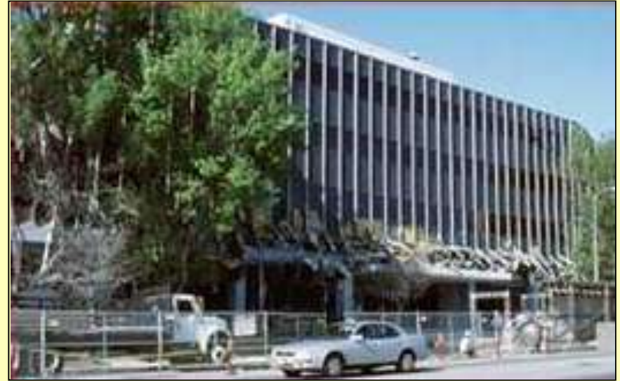
Concrete posts could not withstand the shaking and collapsed allowing upper stories to crush second floor inhabitants.
