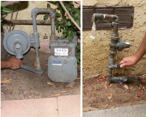
Shut-off Electricity & Gas if fire or leaking gas. Shutoff Electricity & Water if a water leak.
